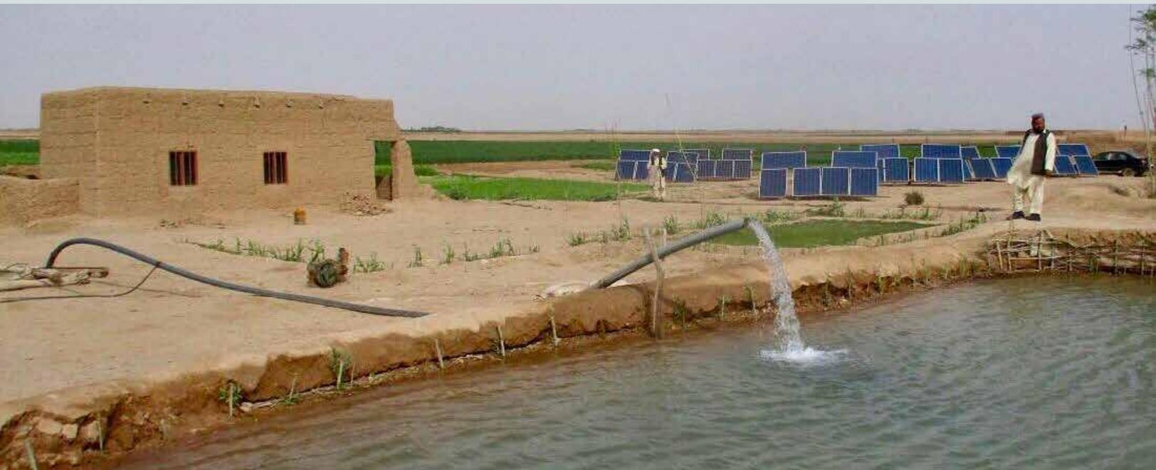
*Figure 4: A farmer examining his solar powered deep well and reservoir in Helmand*
